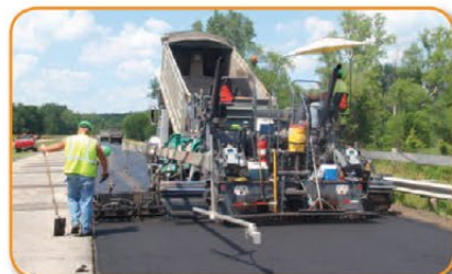
Ohio DOT, SR-13, USA
